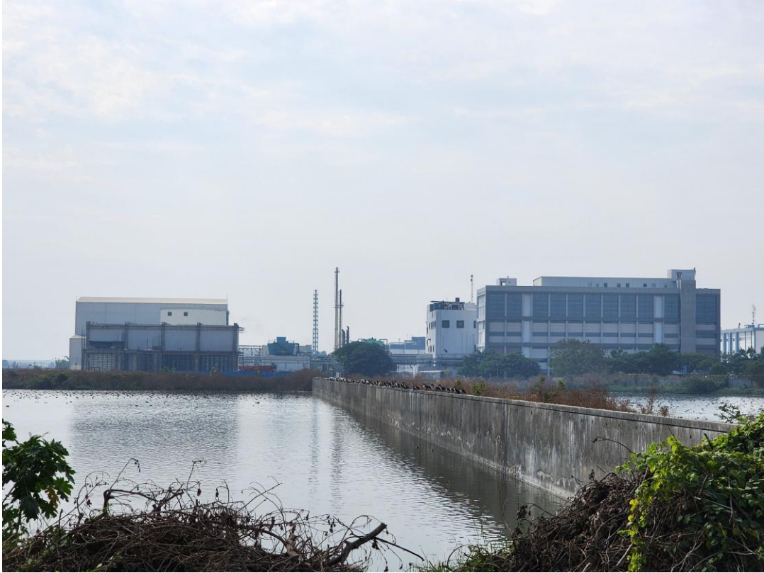
Boundary wall around the wetland prevents outflow
